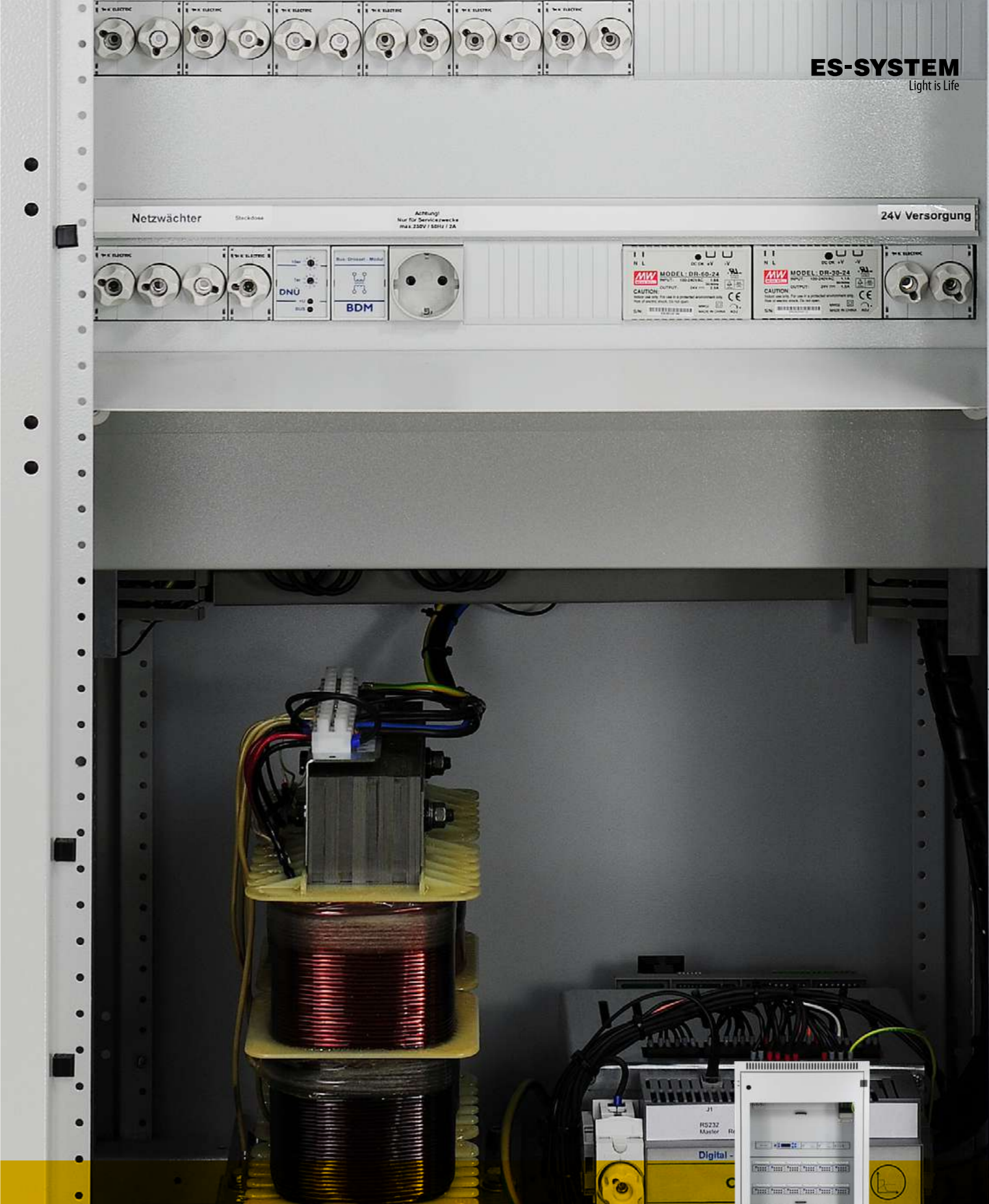
Bateria centralna ES-NET ES-NET central battery
